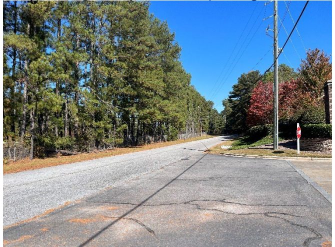
View northeast along Brighton Hill Road
