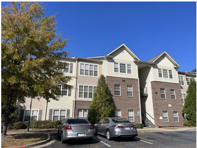
Subject's exterior and typical surface parking
