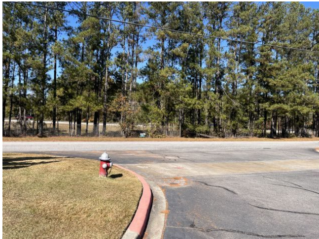
Brighton Hill Road north of the Subject
